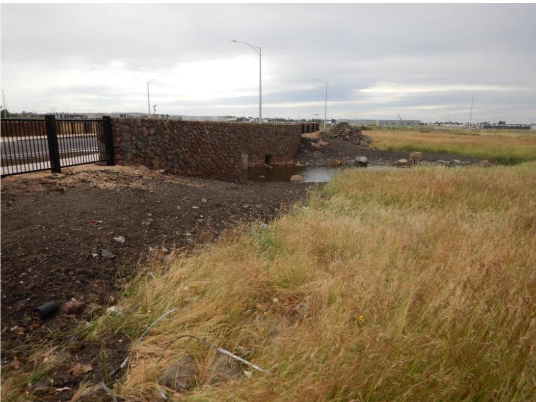
Photo 4: A pile of rocks has been left after works on the crossing of Scanlon Drive (far side of the creek)
